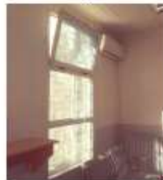
Figure 3. a) Windows in counter area, b) Windows in reception hall, c) Maximum opening of window
