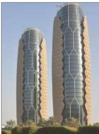
Figure 3.19. Al Bahr Towers. Source : Cilento (2012).
