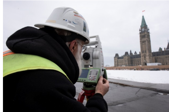
Figure 5.13. Surveying the exterior of the Centre Block in February 2020 (Source: Public Services and Procurement Canada, 2021)
