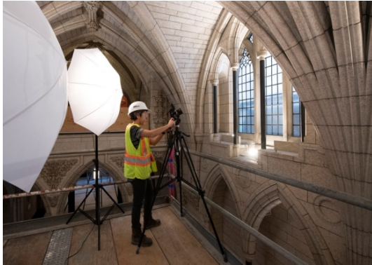
Figure 5.12. Photogrammetry: in February 2020, a worker takes photos of the Hall of Honour (Source: Public Services and Procurement Canada, 2021)
