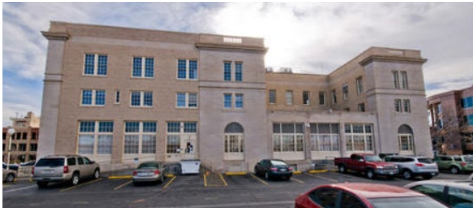
Figure 5.3. North Elevation before renovation (Source: Westlake Reed Leskosky, 2019)
