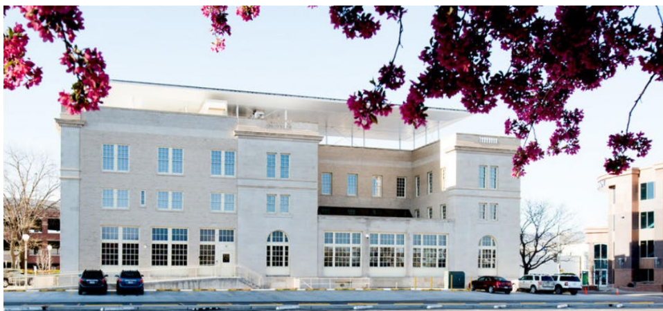
Figure 5.4. North Elevation after renovation and installation of photovoltaic array at canopy (Source: https://www.aiatopten.org/node/367 )
