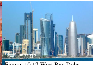
Figure 10.17 West Bay Doha. Source : Salama, A. (2012)
