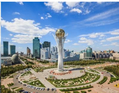
Figure 10.13 tour Bajterek, Astana Kazakhstan, 2002, Akmurza Rustembekov Source : Yussupova, A.A. et al. (2017), op.cit. p599.
