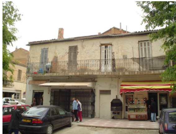
Figure 34 Hara Belkhir (Rue Abbane Ramadan)
