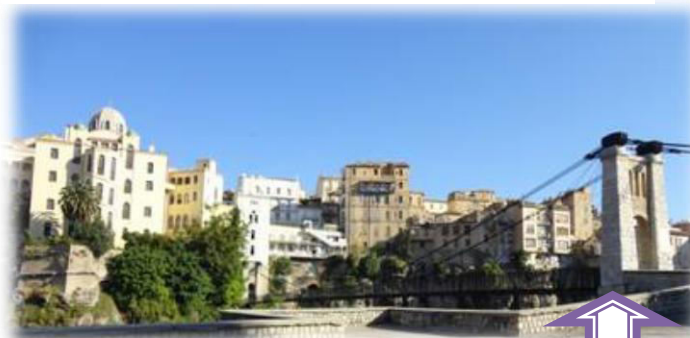
Figure 43: La passerelle Mellah Slimane
