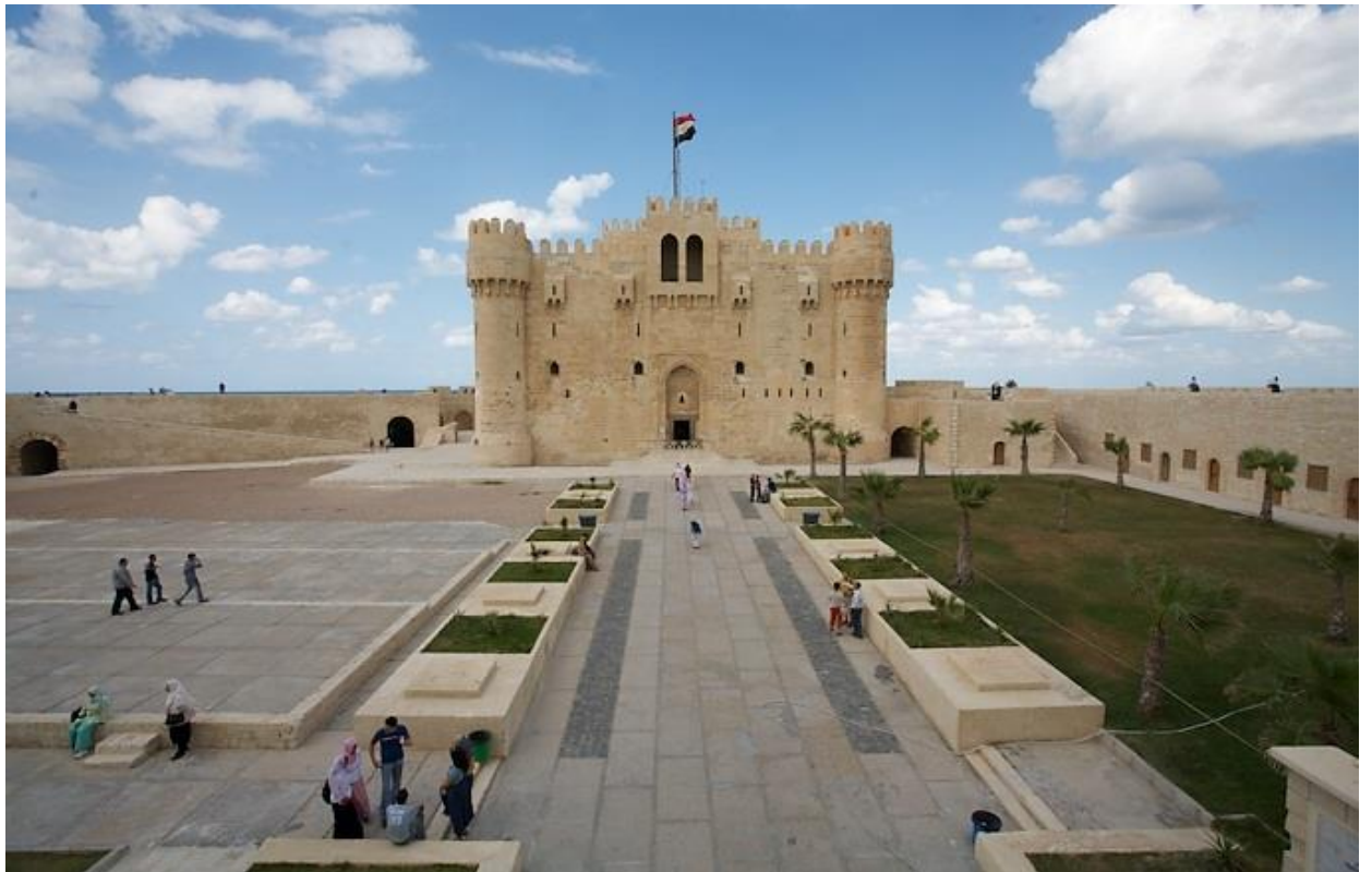
Figure 35. Citadelle de Qait-bay, source : http://en.wikipedia.org/wiki/Citadel_of_Qaitbay
