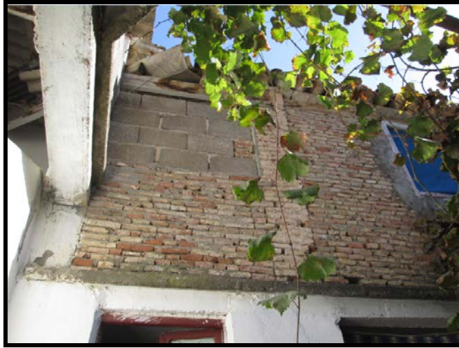
Photo 4.11 : Incorporation du parpaing.
