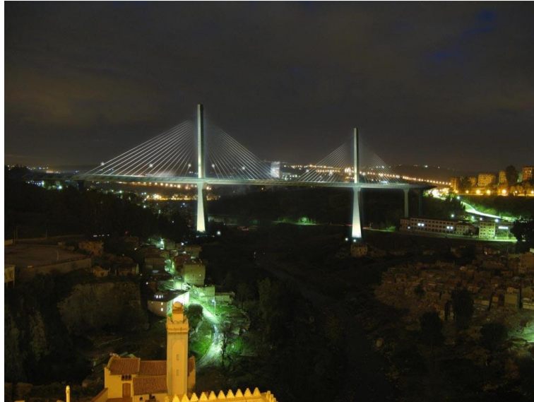
Figure 6.31 Viaduc de Saleh Bey.
