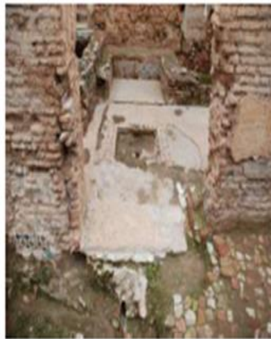
Fig. 6: The condition of the palace before the operation in 2009.
