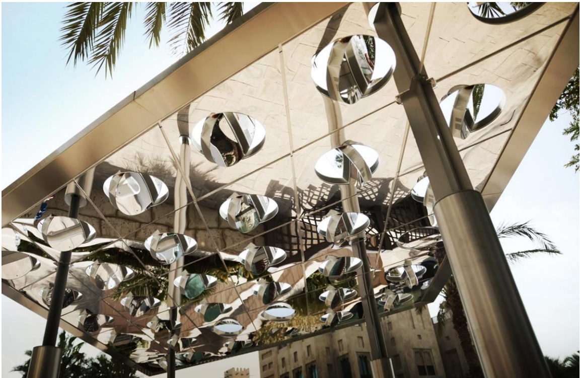
Figure2.21: “Sun and Shade”, a digitally–controlled cover that combines the solar power generation with cooling of outdoor areas (Carlo Ratti-2017-)
