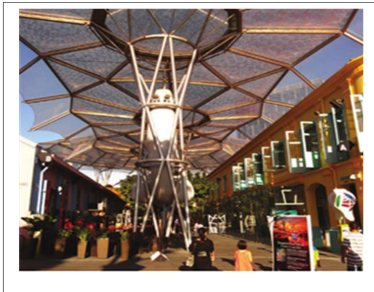
Figure 2.16: Transparent and semi-transparent canopies in Clarke Quay, Singapore. Source: ImSik Cho et al (2015)
