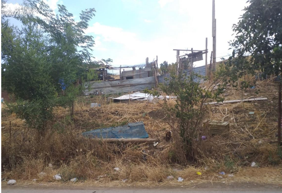
Figure 5.42 : Construction nuisible, Constantine
