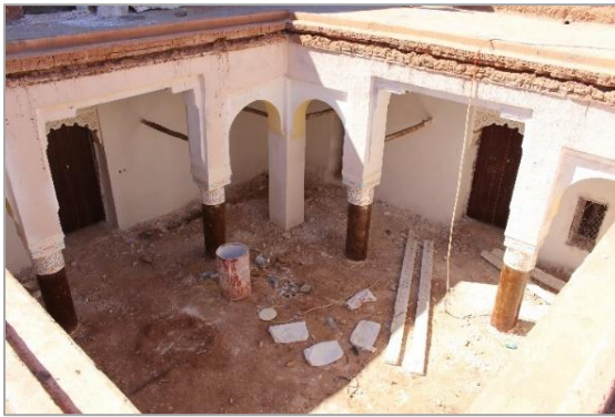
Patio a 12 poteaux
