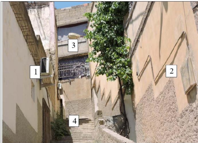
Figure 7a: The regularized settlement Lalaouia Source: Authors, 2019 1- Electricity (airconditioner) 2- Gas 3- Public lighting 4- Stairs
