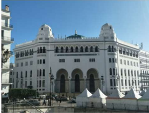
Figure 5. The big post office in Algiers (Voinot and Tondoire 1909-1913) (Photo Authors, Nov.2019)
