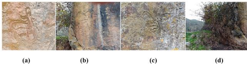
Plate 4. Photos showing the condition of the engraved rock: (a) 100 prehistoric rock engravings; (b) traces of incineration soot on the rock; (c) fungi covering the engravings; (d) weeds invading the rock
