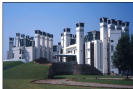
Figure 1. 28: Centre de recherche de Torrenet (Source: Website, http://archnet.org )
