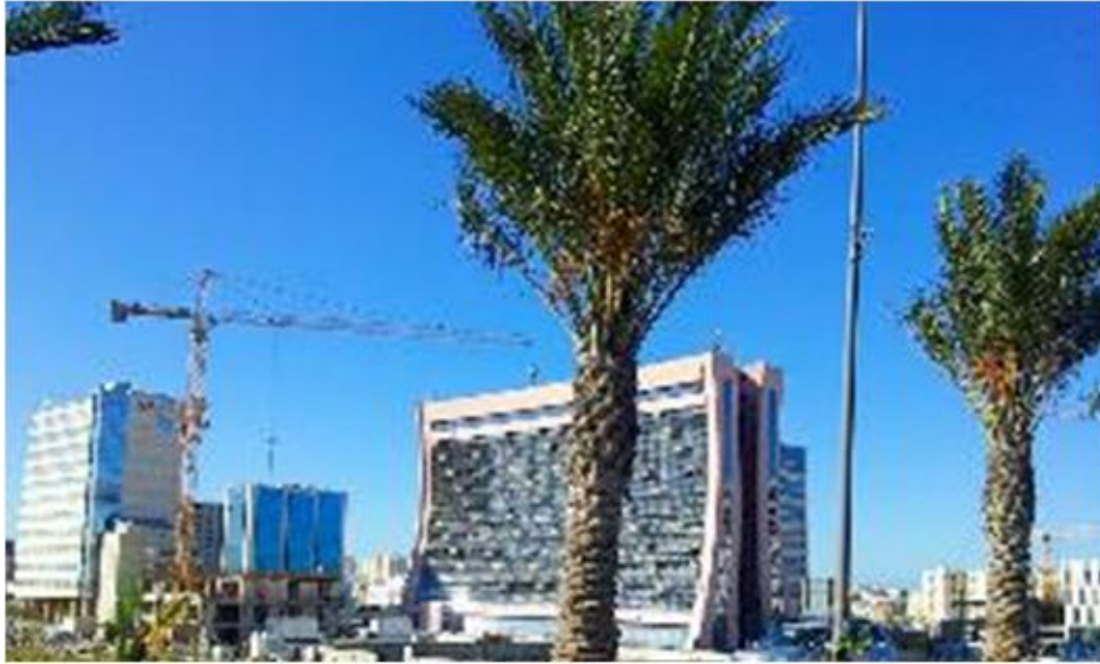
Figure 3: The Business District In Bab Ezzouar
