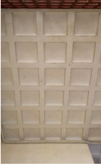
Figure IV-33 Plancher caisson, Climat de France, Alger
