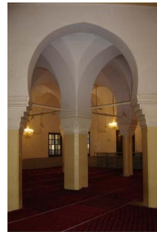
Figure 4.64. Piliers et colonnes supportant la coupole centrale. (source : Benbella, 2008)
