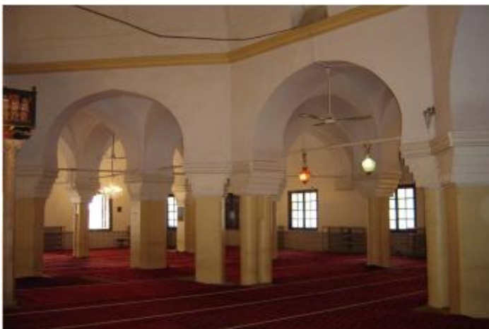
Figure 4.64. Piliers et colonnes supportant la coupole centrale. (source : Benbella, 2008)
