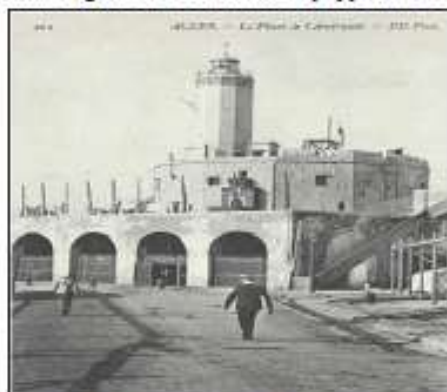
Figure 12. Borj el Fenar, current lighthouse of the Admiralty, Algiers. Source: (ANSS Patrimoine Algérie, 2013)
