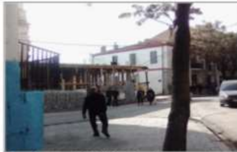
Figure 3. Demolition of old building And reconstruction of a facility
