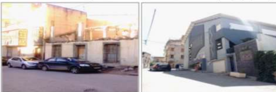
Figure 2. Mutations across the downtown, Demolition of an old building, and reconstruction of a new, more modern one, Source, Bensakhria 2016 and 2022
