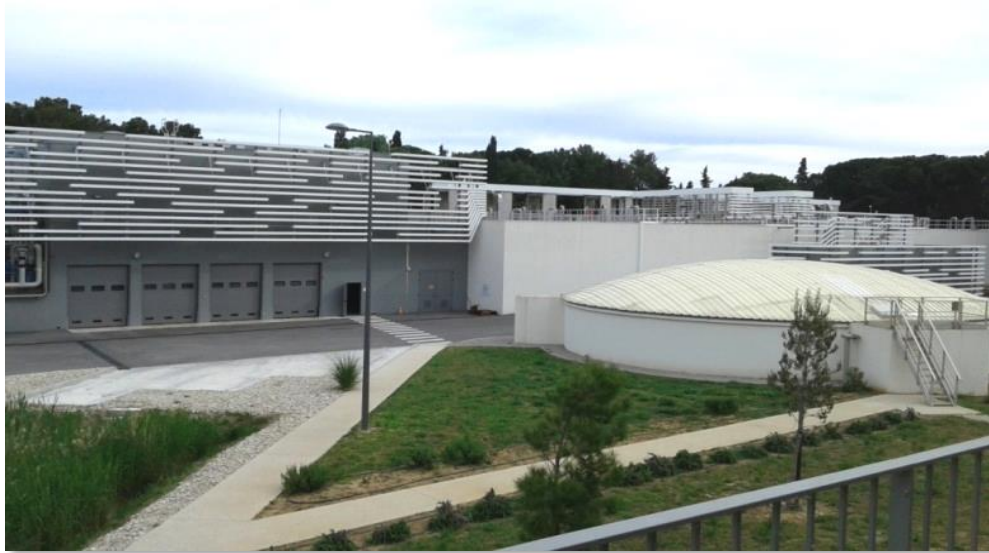
Figure III.11 : Station d'épuration à membrane de GRANDE MONTE, France.
