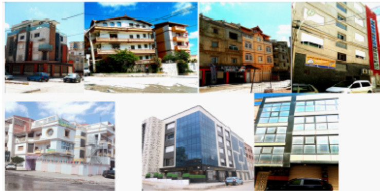
Figure 6. Exceeding permitted heights and misuse of functions
