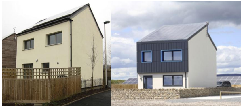
Figure 4. 1 Projets NZEB: a. Lime house (2011), b.Solcer house (2015). (Source: Coma , 2020)
