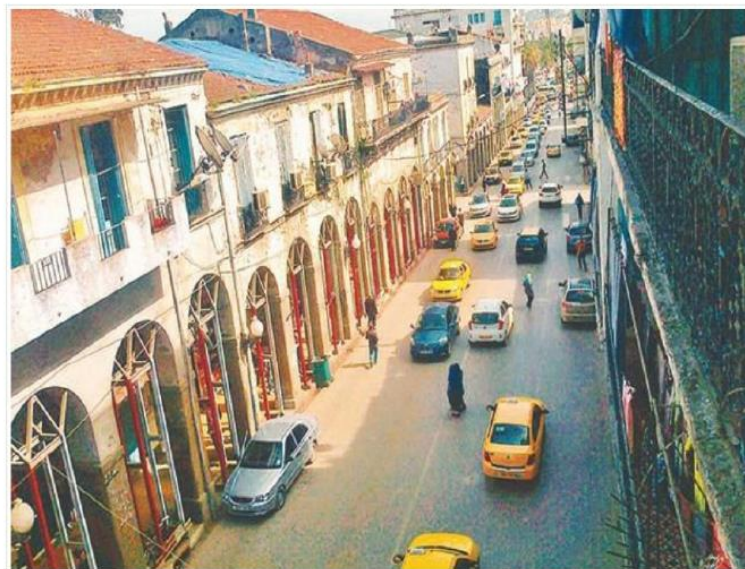
Figure 8. Stabilisation of the main boulevard arcades
