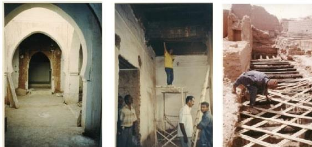
Fig. 6. The rehabilitation works in houses and paths
