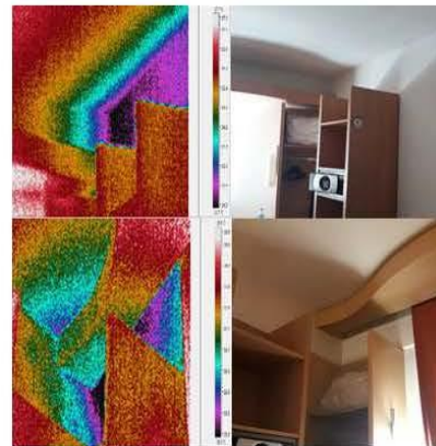
Figure 6. Infrared thermography of interior Rooms.
