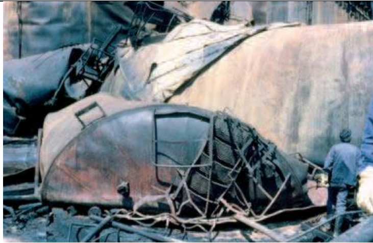
Photo 3: Hydrocarbon tank after an internal explosion.
