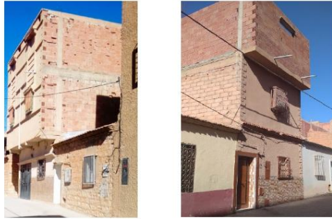
Photos 1-2: Create vertical extensions by adding one or more floors Source: Researchers, Residential samples, Qananineighbourhood. 2022
