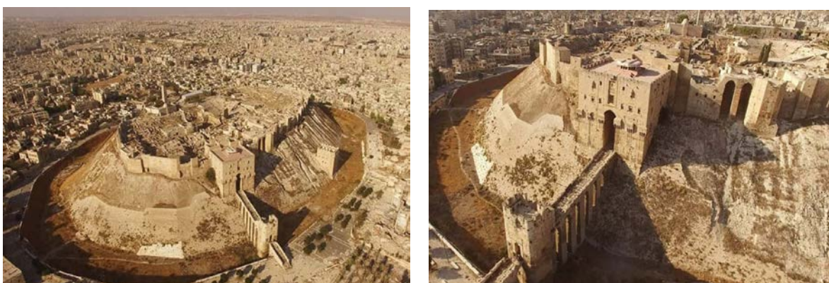
Figure 2.21. La citadelle d'Alep. Source : https://madainproject.com/citadel_of_aleppo
