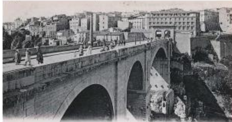
Figure 4. The New Bridge and Gate of El Kantara - In 19XX.
