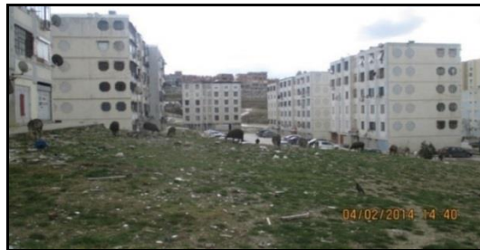
Figure 13. City of 900 dwellings; a no man's land where urban practices and other rural practices intermingle.
