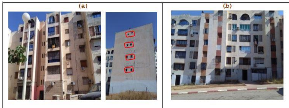
Figure 14. (a) Facade of housing type PRH variant 3 Transformations with creation of openings for sanitary facilities, (b) Facade of housing type PRH to NU8 variant 1, 2 shows the different transformations in facade
